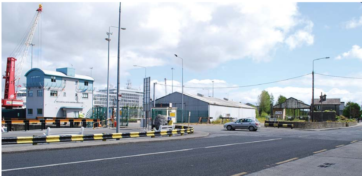
Figure 9.1 Existing Foynes Port Entrance
