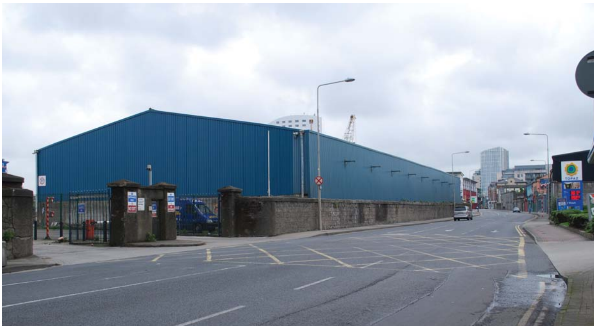
Figure 9.7 Existing Main Vehicular Entrance and Warehouse
