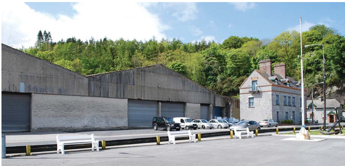
Figure 9.3 Existing Warehouse Buildings
